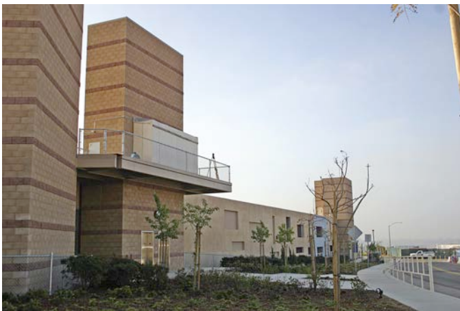
The new parking garage was opened in Dec 2007 and provided many new and larger spaces (view to south from orthopedic office).
