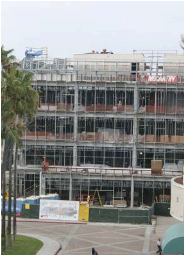
Construction well underway May 2009 (view to south from orthopedic office)
