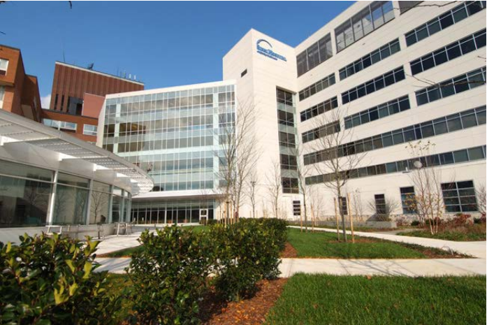
Sinai Hospital of Baltimore
