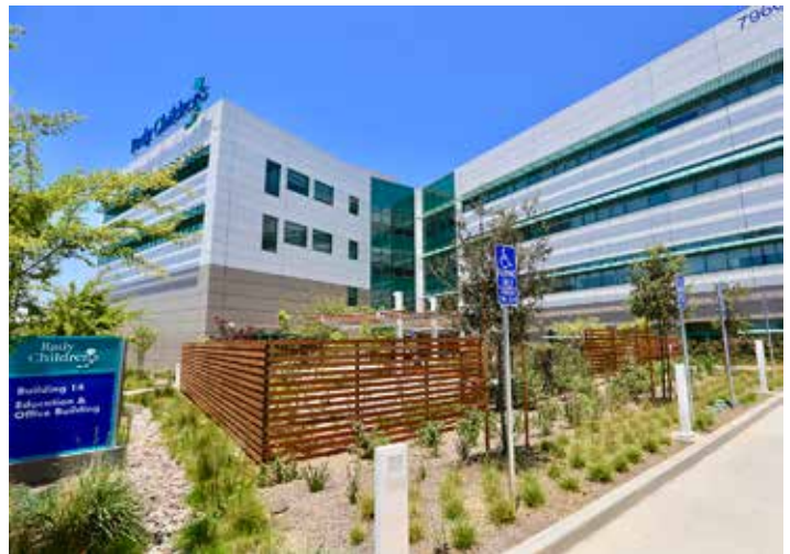
Our new Education and Office Building (EOB).
