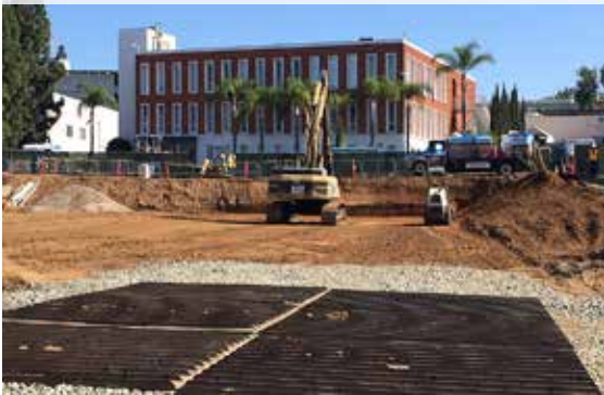
Early excavation (just south of “gait lab” building)
